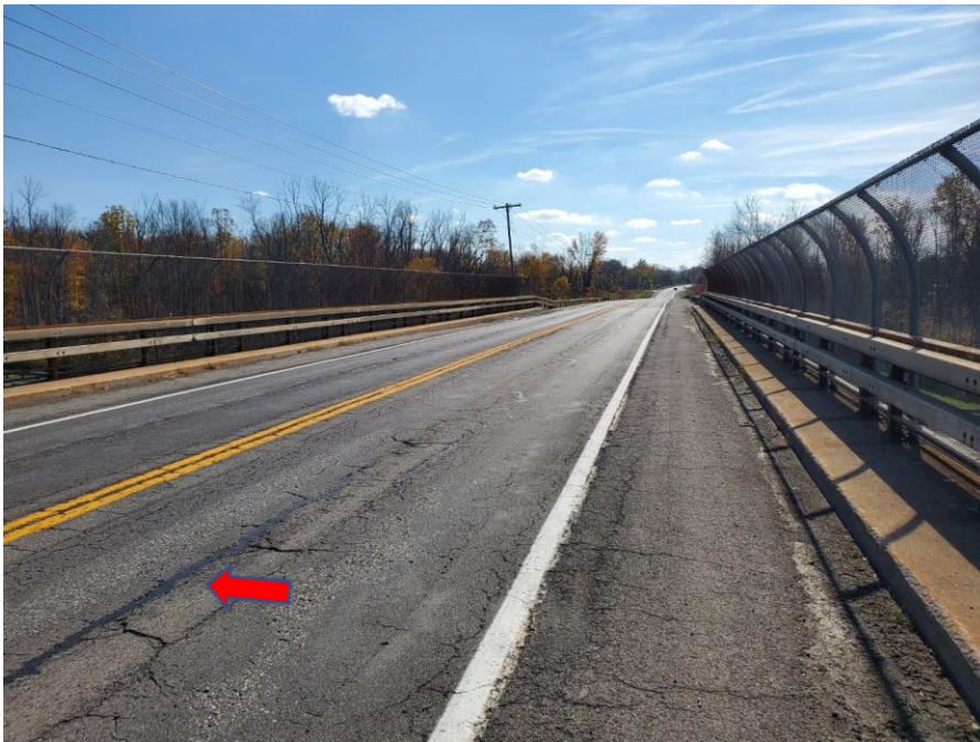
Photograph 4 – View of non-ACM black crack sealer on bridge road surface (ACM-7 & ACM-8)
