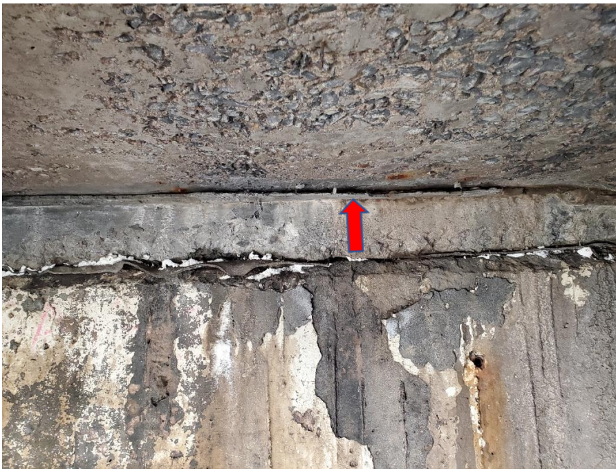
Photograph 3 – View of non-ACM gray/white concrete with fibers south end underside of bridge (ACM-5 & ACM-6)
