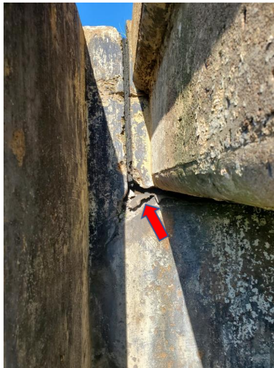
Photograph 8 – View of non-ACM grey bridge bond breaker at north end of bridge (ACM-14)
