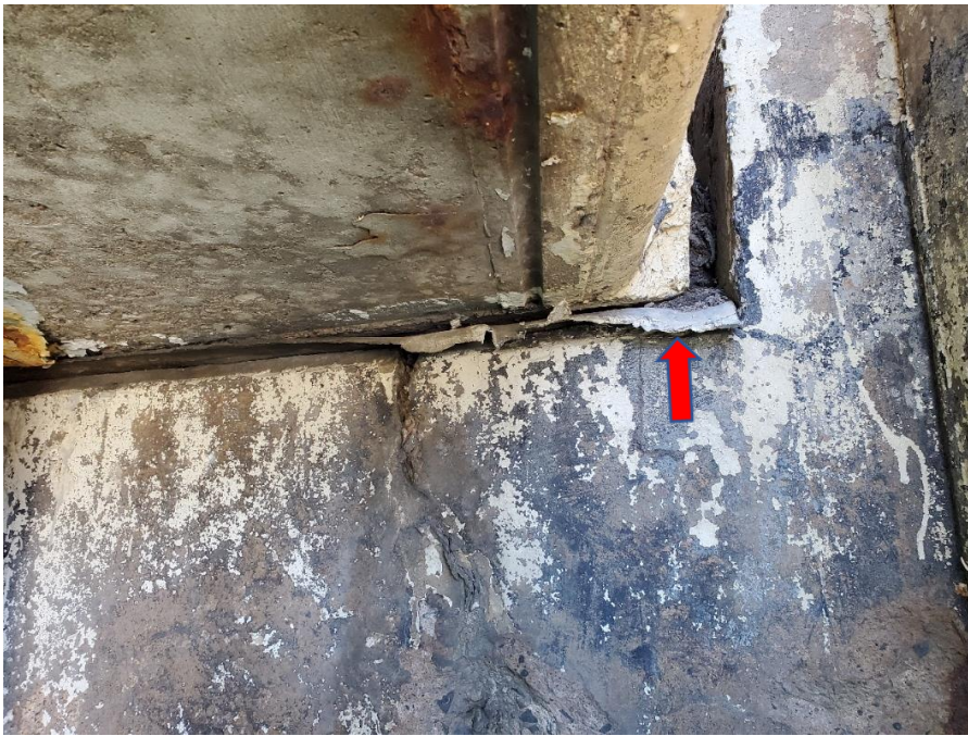
Photograph 7 – View of non-ACM grey bridge bond breaker at south end of bridge (ACM-13)
