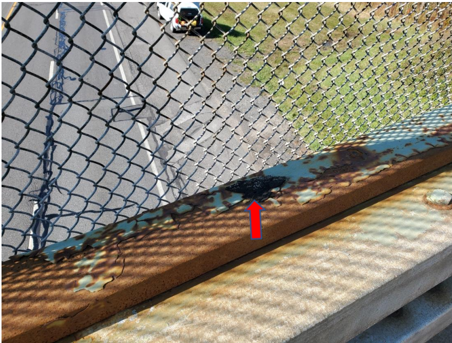
Photograph 5 – View of non-ACM black tar sealer on bridge guardrail (ACM-9 & ACM-10)
