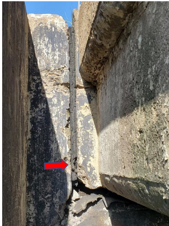
Photograph 6 – View of non-ACM black expansion joint at north end underside of bridge (ACM-11 & ACM-12)
