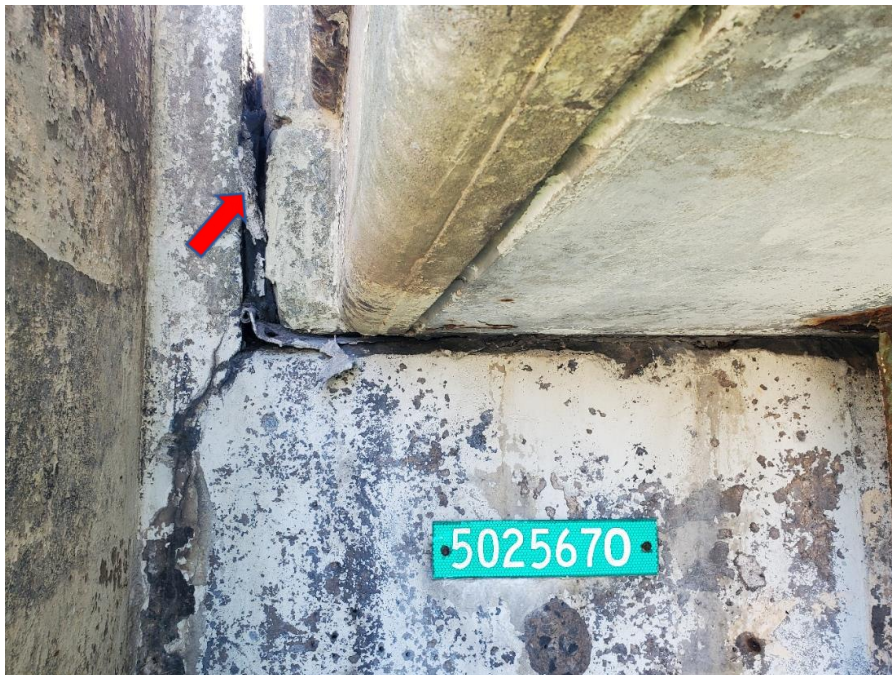
Photograph 2 – View of ACM black expansion joint on south end underside of bridge (ACM-3 & ACM-4 ) – Identified as asbestos containing.
